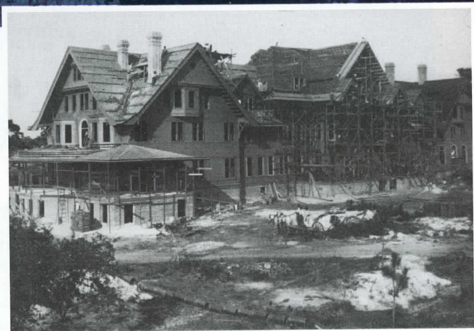
The Bellevue Mido in her fledgling, construction-filled days.
